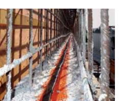
**PENEBAR PRIMER** is applied first to the area where the waterstop is to be placed. It is quickly and conveniently applied at the job site by a simple brush application.
