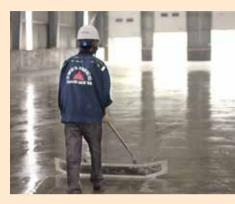
PENESEAL FH sealer goes on with just a single coating, reducing floor maintenance and repair costs.
