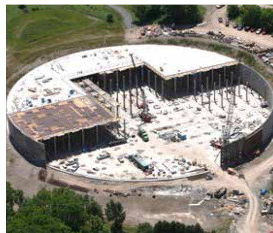
Working to a budget: OCWA Eastern Reservoir, USA PENETRON ADMIX was used in the ready-mix concrete to meet a tight project budget by saving man-hours, eliminating the need for membranes and coatings, and providing superior performance.
