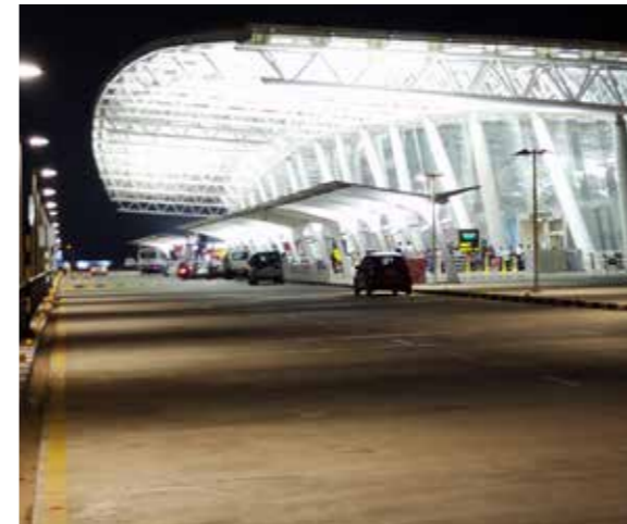
Chennai International Airport, India
