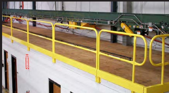
MECHANICAL SERVICE AREAS
