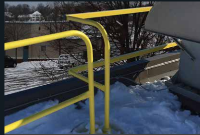
IN-LINE PARAPET RAILING
