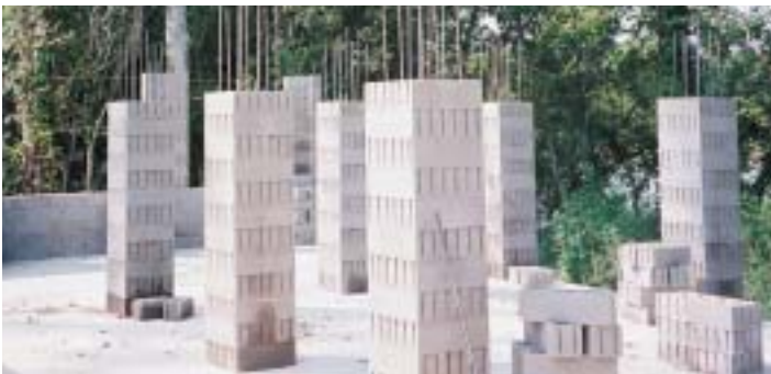
VOBB columns for the porch and garage
