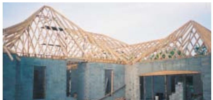
Front view with rafters
