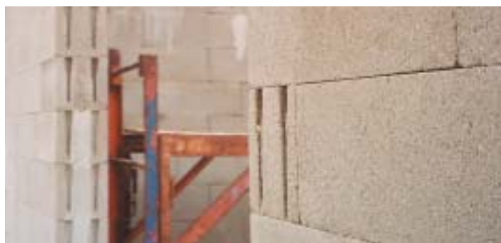
Up close view of dry-stacked VOBB
