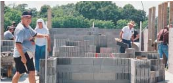
A level must be used to have a straight wall
