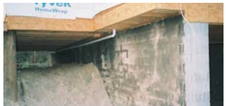
VOBB blocks being used for a basement
