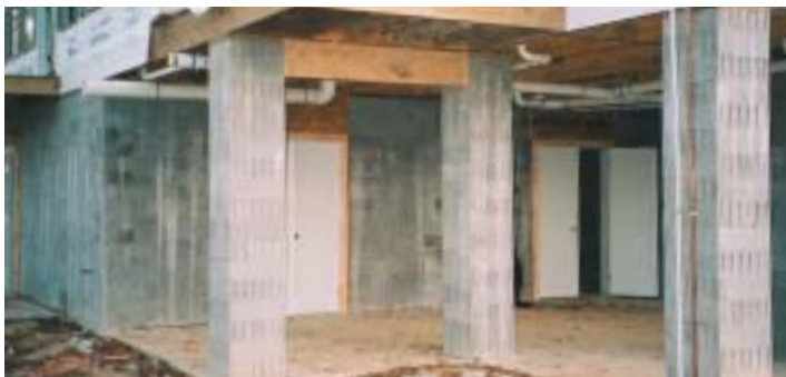
VOBB walls and columns
