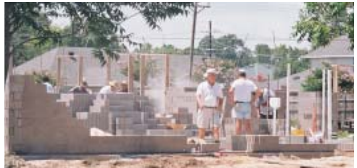
The exterior wall is dry-stacked
