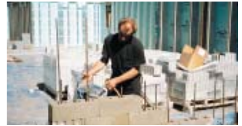
Spraying in water as needed and mixing inside the cavity
