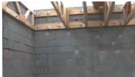
Trusses for second floor
