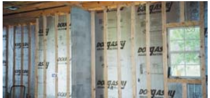
Insulation is installed on the exterior walls
