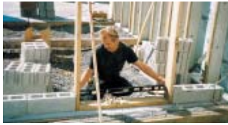
Use a level to set the doors
