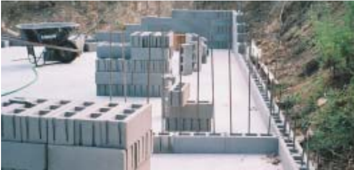
Start with the first row and dry-stack a corner
