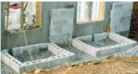
Building a window well
