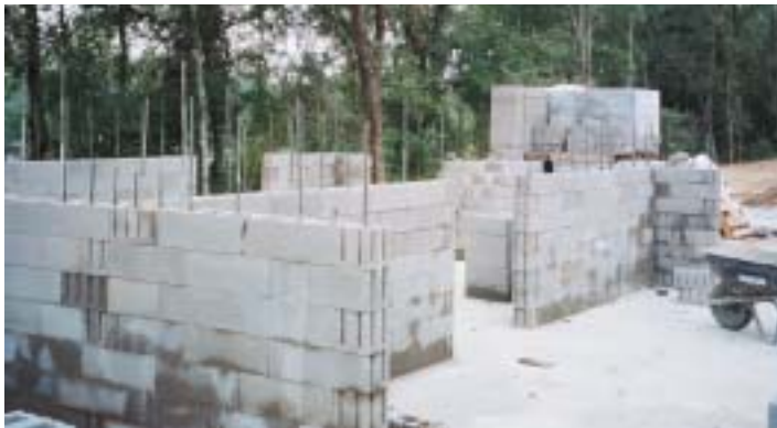
A VOBB wall in-progress
