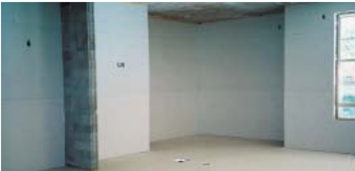
The drywall is installed directly on the VOBB
