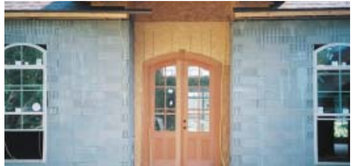
Front entrance before the columns are built
