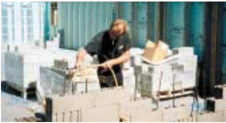
Wetting the blocks FIRST
