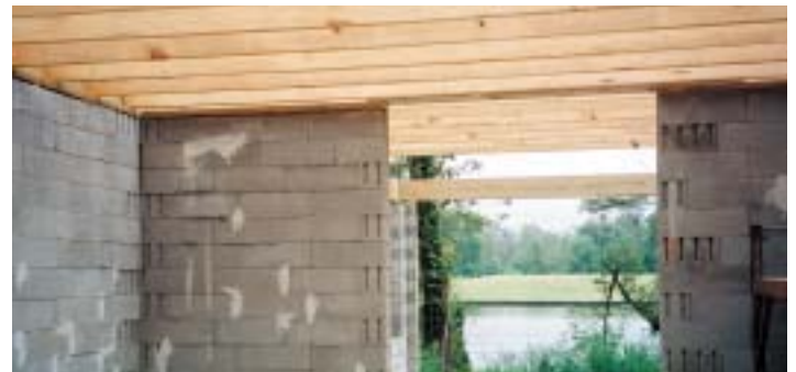
VOBB with the trusses up
