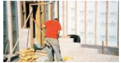
Working from the door frame
