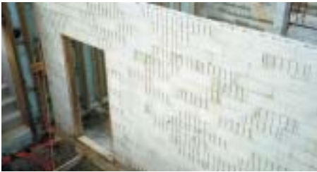
A whole wall viewed from the top
