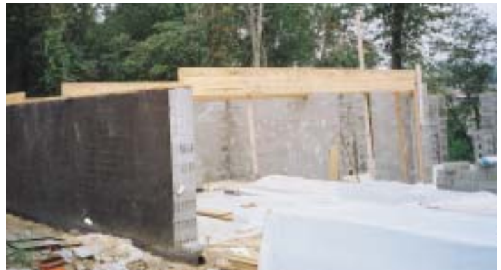
A VOBB basement wall on the river
