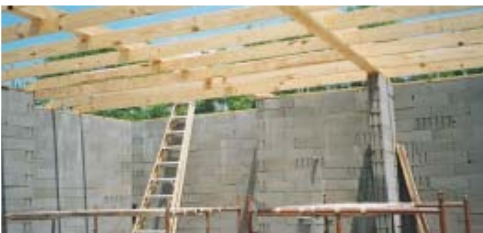
Rafters installed as viewed from the interior
