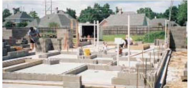
The corners are dry-stacked first
