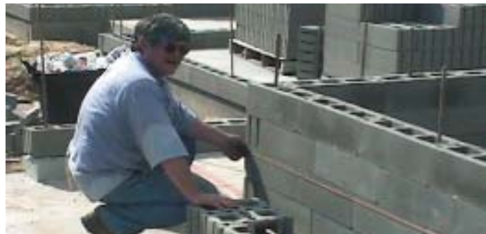
Use a string for the middle between the corners
