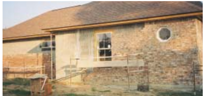
The brick is put up on the exterior
