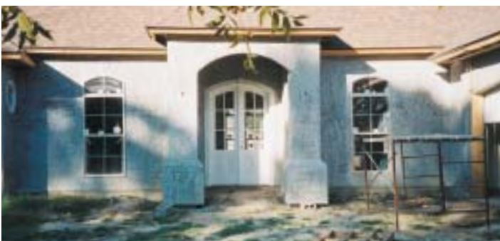
The front columns ready for stucco application
