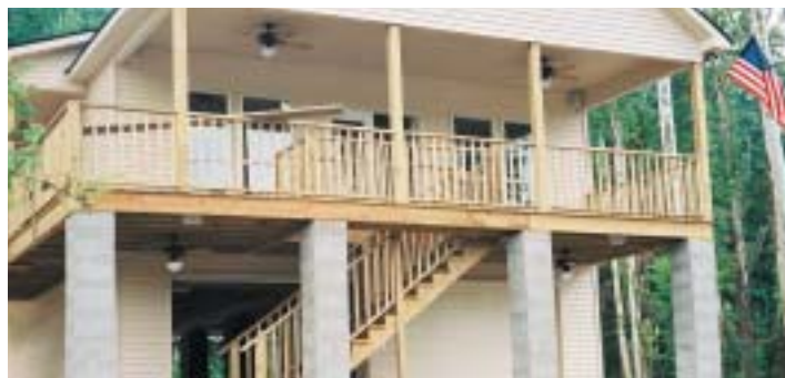
Facing the river with 12" VOBB columns
