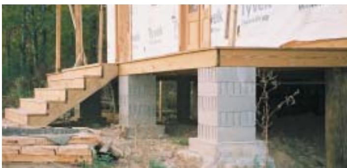
VOBB blocks used for the porch support
