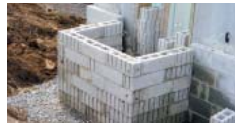
Window well completed
