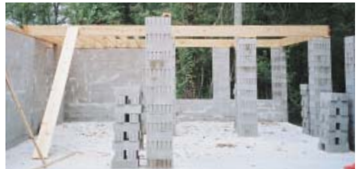
Trusses being put up for the first floor
