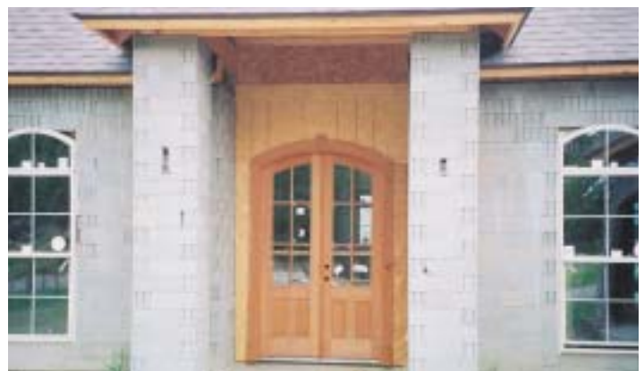
VOBB blocks being used to build columns
