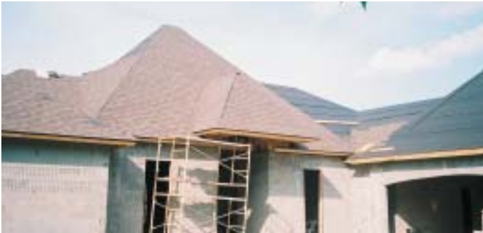
The roof is installed
