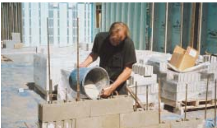
Pouring in the dry concrete mix directly into the cavity
