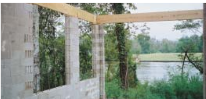
VOBB wall ready for the windows
