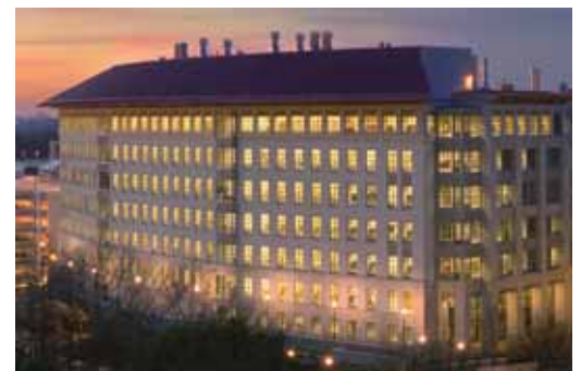
Whitehead Biomedical Research Building Atlanta, Georgia LEED Certification — Silver
