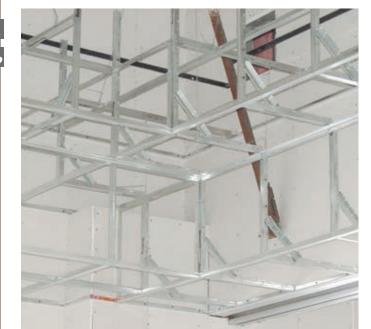
A faster, easier, better way to frame drywall soffits; designed to significantly reduce time and labor associated with cutting and measuring.\*
