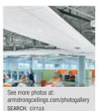
These medium-textured panels, with scored plank visual, provide the noise reduction and sound blocking of Total Acoustics® performance.
