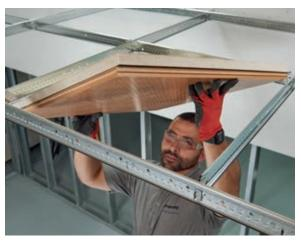
WoodWorks® Tegular ceiling panel with Calla® 2820 acoustic infill panel for Total Acoustics® performance
