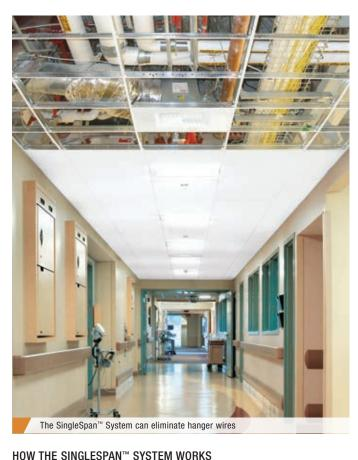
Reduces or eliminates hanger wires for faster, easier installation in crowded plenum spaces
