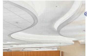
This extruded aluminum perimeter trim is a solution for use as exposed custom decorative trim with suspended panels or drywall.
