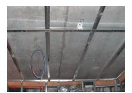
QUIKSTIX™ Drywall Grid System with Locking Pocket Main Beams
