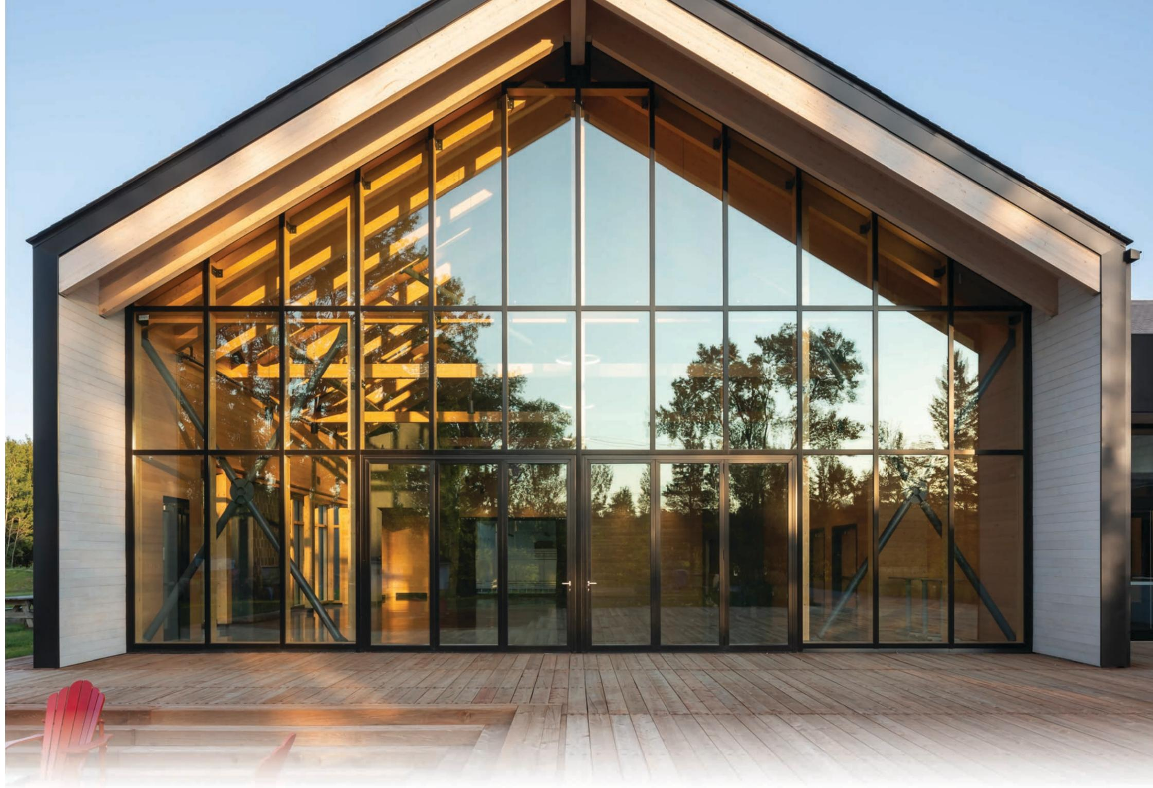
All Unicef Architectural Timber Curtain Wall mullions come fully assembled with all anchors and membranes
